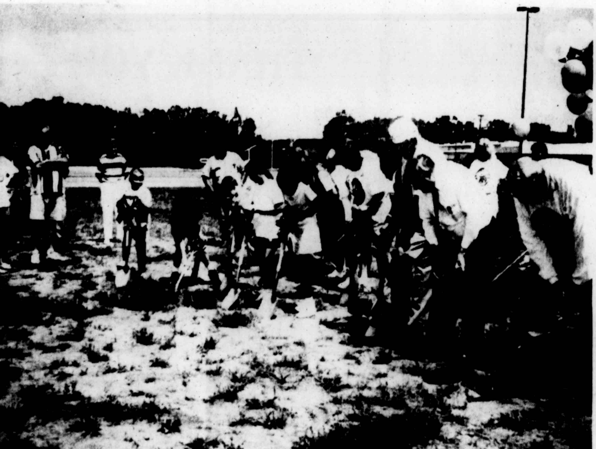
GROUND BREAKING ceremonies for the new branch of Bank of Ripley on Highway 51 By-Pass, in front of Wal-Mart, Children enjoyed a sand dig for money. Construction will begin soon.
